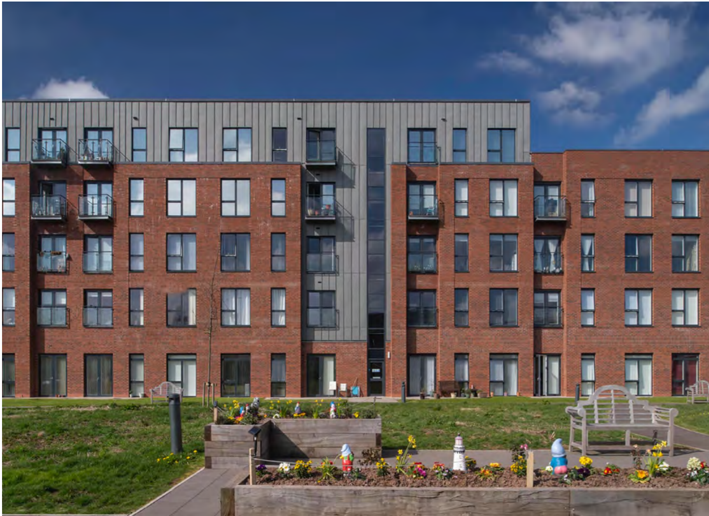
Figure 1 Foundry Wharf, an extra-care apartment building on the edge of St Helens town centre.
